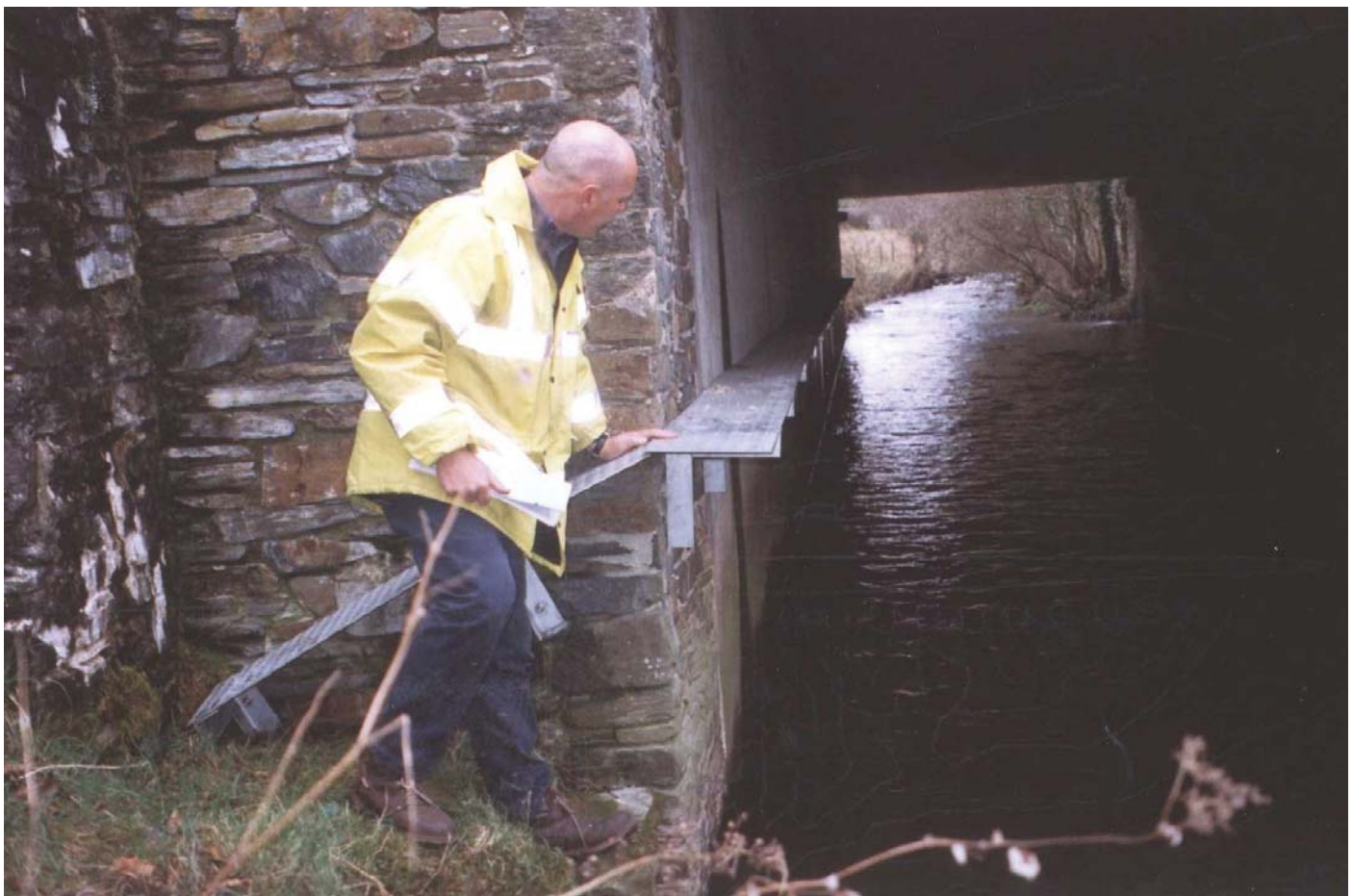
When this bridge was strengthened an otter ledge was incorporated to allow passage during high river flows and stop otters attempting to cross the road. Photo: Kate Stokes
