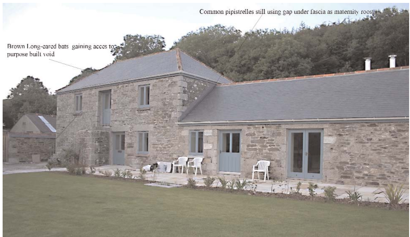
This barn was converted under a protected species licence. Monitoring post-conversion has shown that bats continue to use the building. Photo: Steve Marshall
