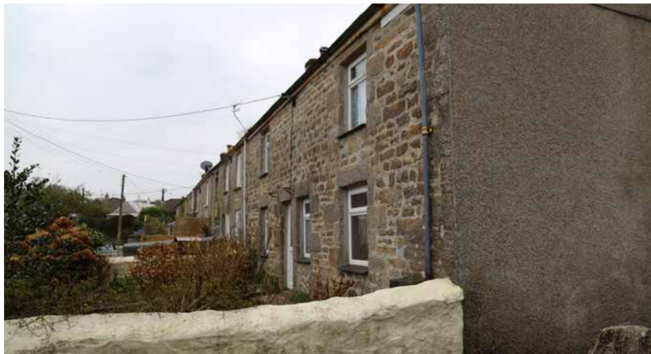
Figure 17: - At Lower Terrace, rubble stone is used, with more mortar. Granite defines window reveals. Note the use of render.
