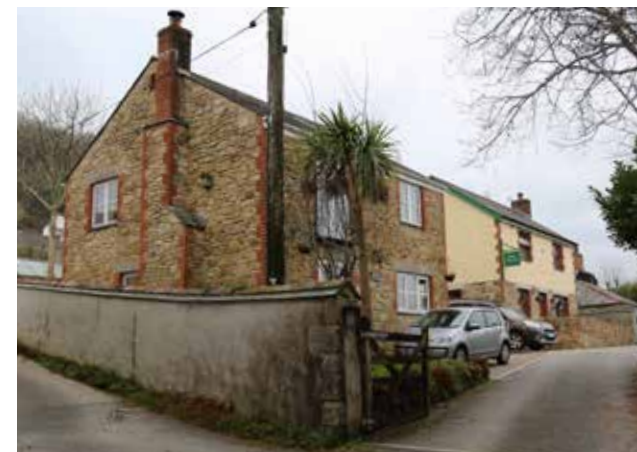
Figure 19: - Stone facade, granite lintel with brick accents.
