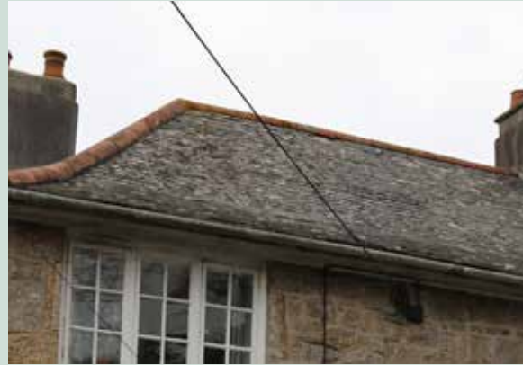
Figure 55: - Scantle slate roof.
