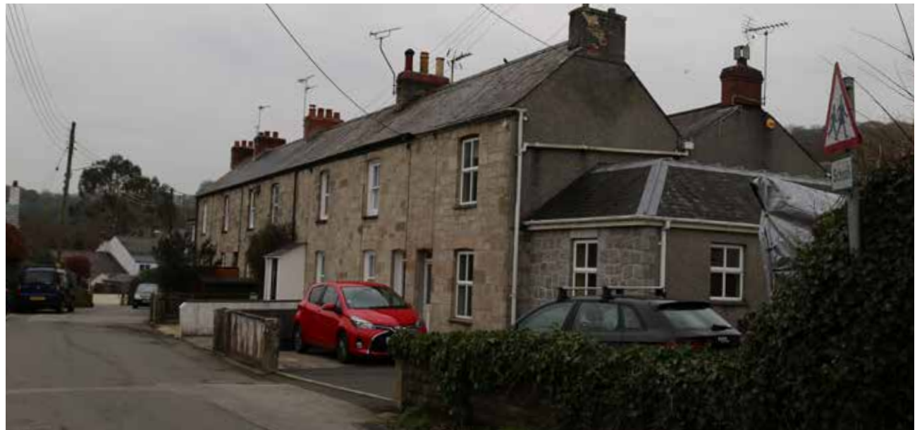
Figure 22: - St Andrews Terrace. Evidence of modifications with porch and extensions.
