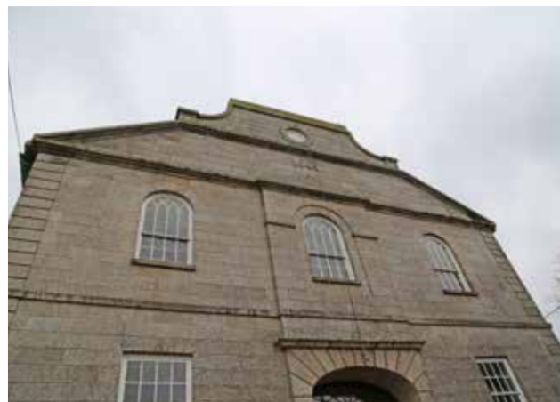
Figure 18: - Granite blocks, central parapet.
