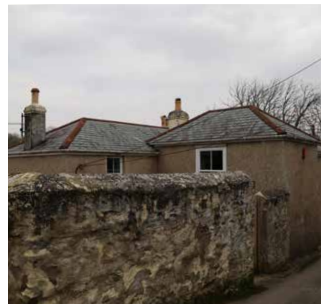
Figure 09: - Weathered stone wall (limewashed) building façade continues boundary. Rough cast render, hipped slate roof.
