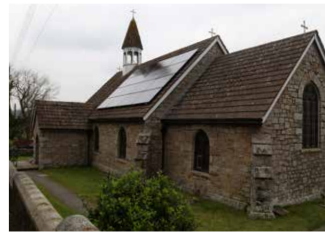
Figure 27: - Gabled stepped roof, with concrete tile.
