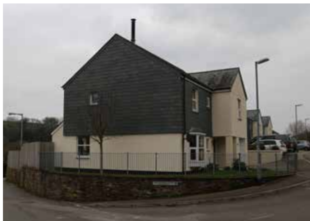
Figure 36: - Slate hanging on gable.
