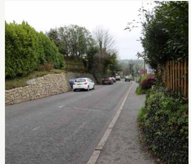
Figure 23: St Michael's Road, upper and lower sides and single sided pavement access.
