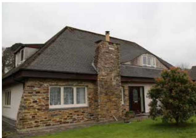
Figure 34: - Feature window, and roof finished in a tile sympathetic to the slate aesthetic.
