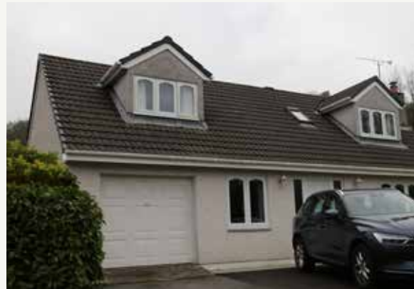
Figure 71: - Simple material changes could integrate this bungalow better with settlement character.
