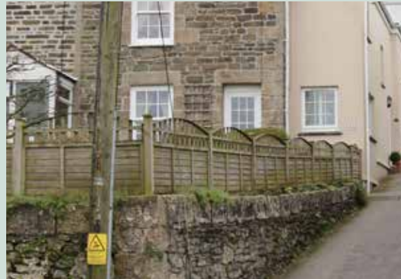
Figure 70: - Example of road facing panel fencing.
