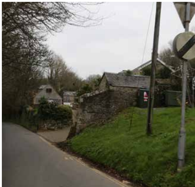
Figure 29: - The Old School House northern elevation and response to levels.
