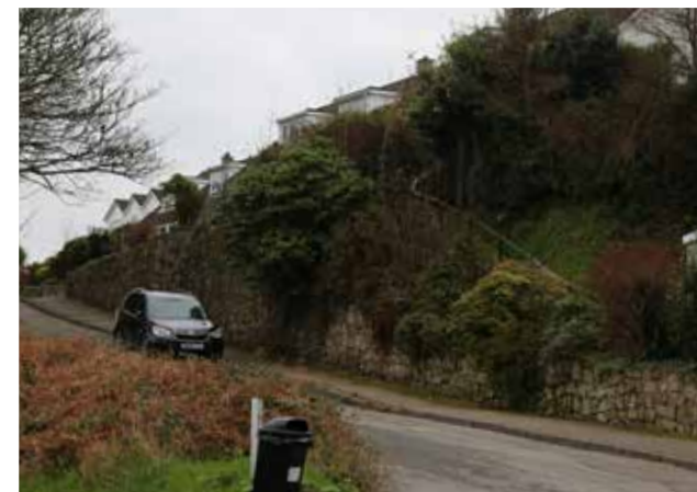
Figure 37: - The approach to Cott Wood as topography begins to rise.
