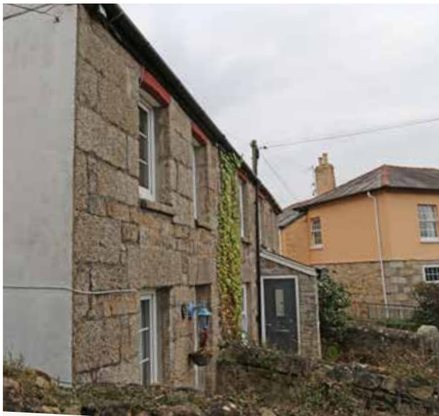
Figure 07: - Contrasting material finishes (rendered gable).
