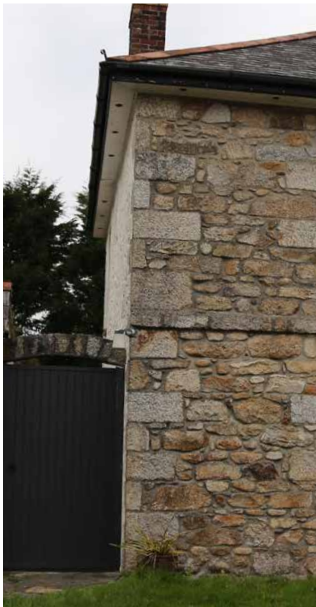
Figure 16: - Roof overhangs at verge, quoin detail and string course.
