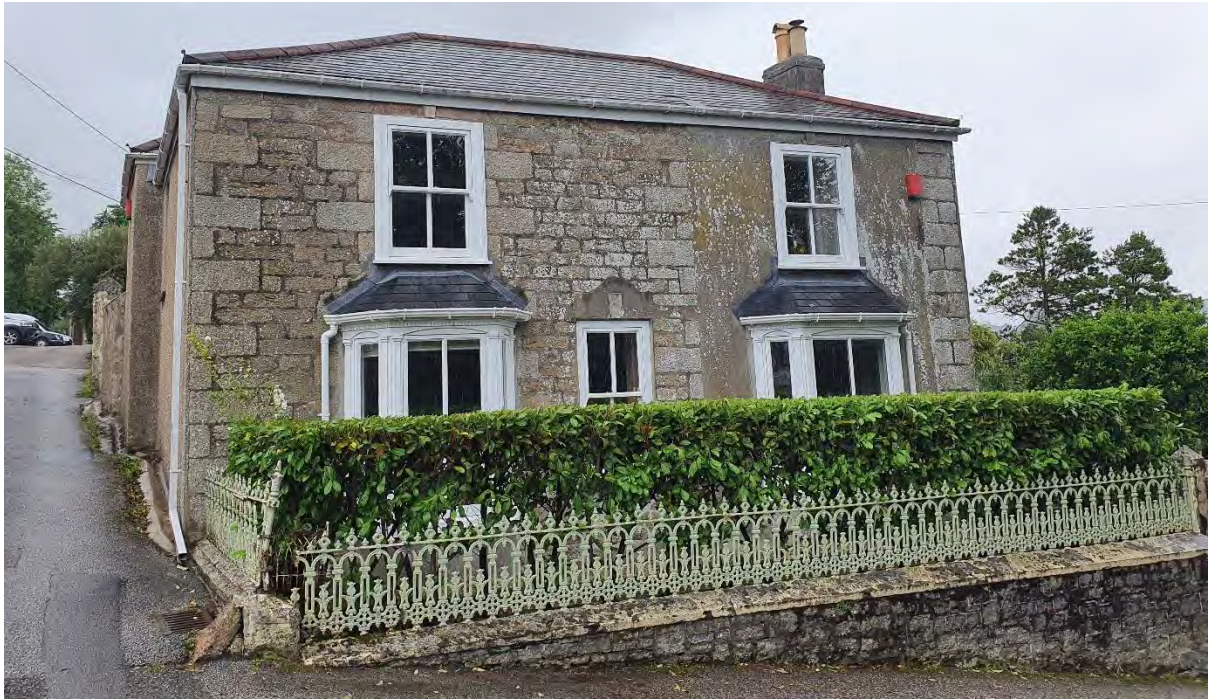
Another substantial house is 14 Commercial Hill, with squared and coursed granite and sharply shaped quoins and generous sized rooms. It was extended and made grander with fine bay windows, porched door and new hipped roof (and a large walled and railed garden) in the mid 19 th century. It stands within a group, including Mill House, that seems to have formed a small higher status quarter, perhaps the homes of more senior employees in the nearby gunpowder or woollen factories.
