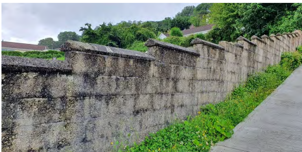
Well designed and executed coped concrete block wall alongside the 20 th century cemetery established on the east side of Rye Hill. While employing early modern materials, it is in tune with the scale and form of earlier Ponsanooth walls retains a sense of local style.
