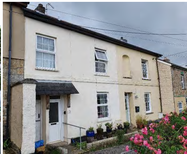
Stucco panels in a pebbledash render at the eastern end of Higher Terrace (the end formerly known as Lemon Terrace) (left) and a pair of stuccoed houses in Eddystone Place, further west in Higher Terrace. Note the arched first floor niche; a feature fairly distinctive of Ponsanooth parish.
