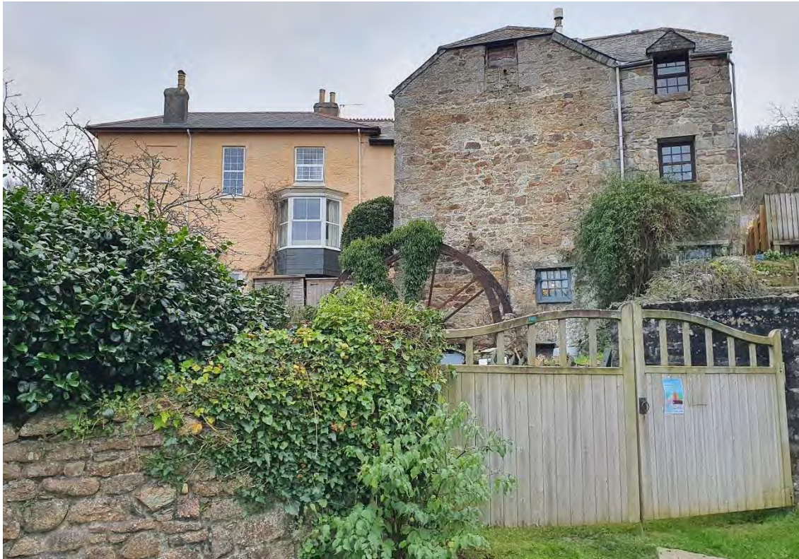
The three-storeyed Tregoose Mill with remnants of a cast iron rimmed waterwheel on its near north wall. Mill House, one of Ponsanooth's more substantial houses, stands to its rear.
