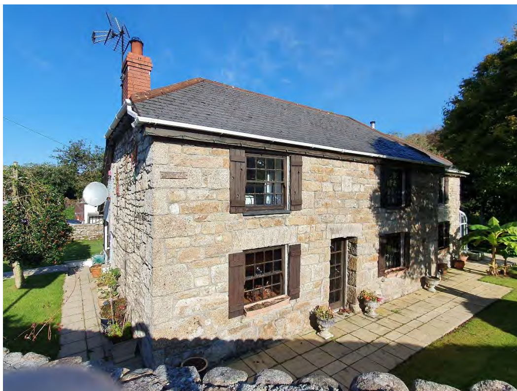
Brook Villa, immediately south-west of Ponsanooth bridge has a datestone (1816) and a style with half-hipped roof, coursed, roughly squared granite rubble and false segmented lintels (scribed onto plain lintels) that indicate a relatively early higher status dwelling. With the Victory Inn it contributed to an impressive group at the early heart of the village.
