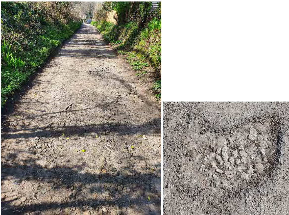
Commons Lane with detail of original granite metalling
