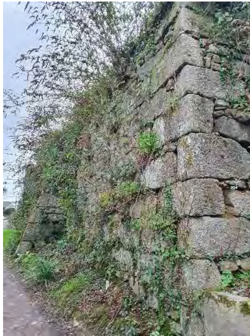
The buttressed revetment of the millpond immediately north of the chapel.
