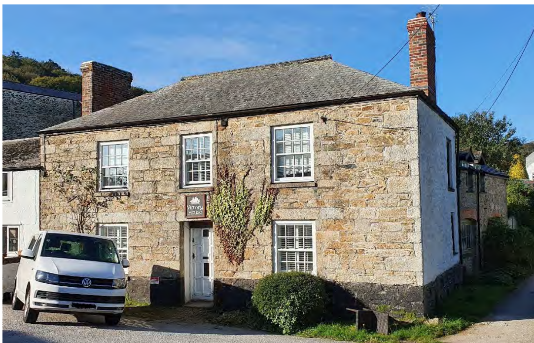
The Georgian public house, the Victory Inn, beside the main Redruth-Penryn road. Roughly coursed granite rubble with strong shaped granite quoins and lintels and substantial brick end stacks standing tall from the hipped roof. Possibly the earliest surviving house in Ponsanooth (named from Trafalgar in 1805); among the grandest.
