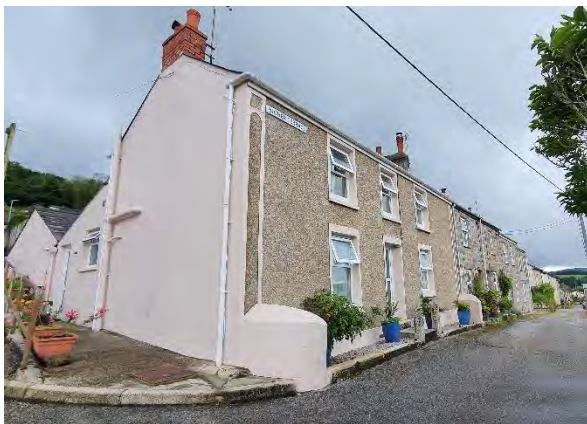
Stucco panels in a pebbledash render at the eastern end of Higher Terrace (the end formerly known as Lemon Terrace) (left) and a pair of stuccoed houses in Eddystone Place, further west in Higher Terrace. Note the arched first floor niche; a feature fairly distinctive of Ponsanooth parish.
