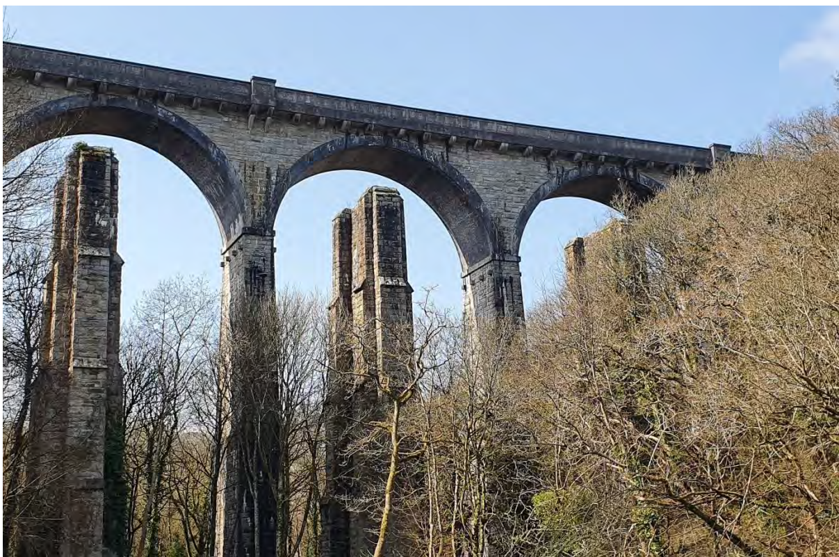
The great viaduct of the Cornwall Railway from the east with piers of the first granite and timber railway viaduct standing in front of the 1930 replacement.
