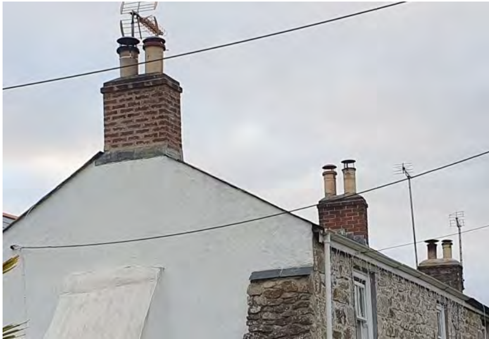
Typical simple Ponsanooth chimney forms with brick stacks with single-course drip moulds and cream ceramic pipes (1-4 Victoria Place)
