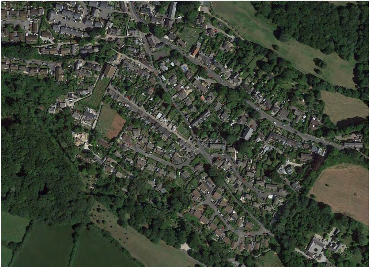
The eastern half of Ponsanooth, again with dense distributions of mature trees and minimal public open ground, aside from the three graveyards. (Google Earth 7/21/2020 eye altitude 660 metres)
