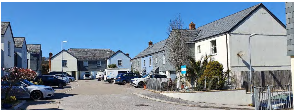
Part of the early 21 st century Trevonnen Road housing estate that draws on Ponsanooth and wider west Cornwall housing styles and materials: gabled slate roofs with simple brick chimneys, slate cladding, render, sash windows, and hooded porches
