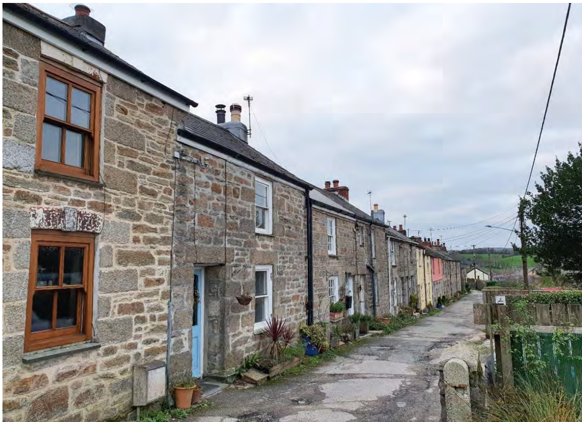
A portion of Higher Terrace's fine line of 19 th century workers' houses and cottages. These form a 'row' of individually constructed buildings, with neighbours rarely sharing the same forms of fenestration (window arrangements), lintels (brick and granite shown here) and chimney styles. Unusually for Ponsanooth, front doors open straight onto the street and their gardens lie across it as well as to the rear of the houses.
