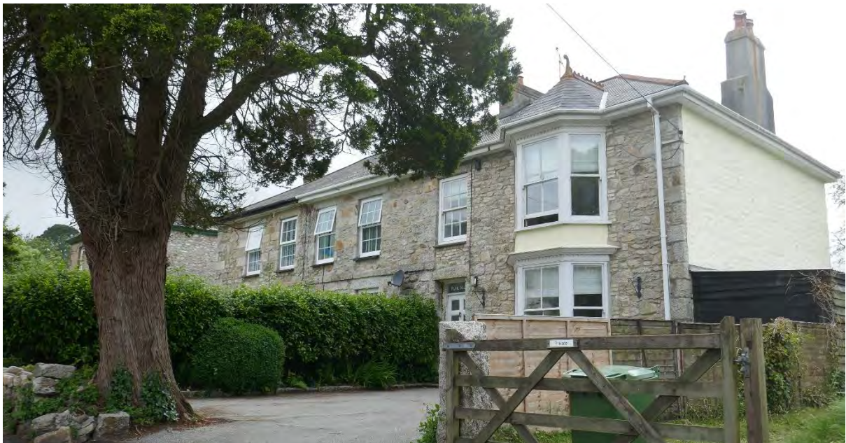
Park Villas and Cottages, two rooms deep, hipped rooves, ornate finishings, and good quality sash windows, form a small 'west end' of Ponsanooth, a gathering of substantial well-built dwellings of the middle Victorian period. Walls would have been stuccoed
