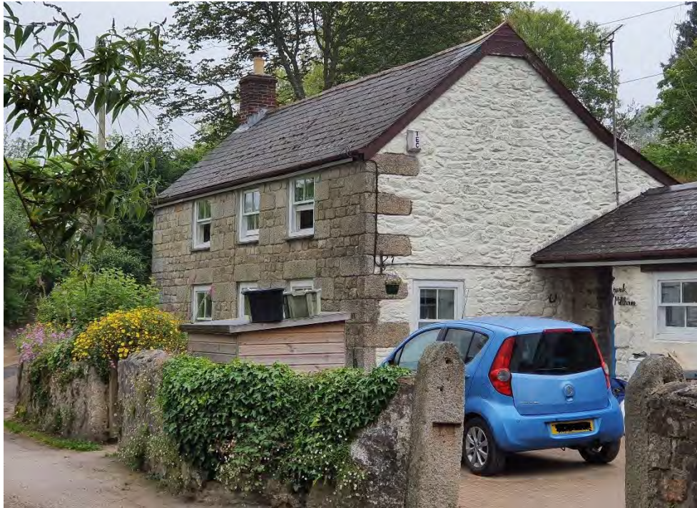
Carrick Millhouse, immediately adjacent to the main millpond, has neatly coursed roughly squared granite on its northern front (but more typical rubble stonework on the now painted gable wall). It may be another relatively early house, perhaps a miller's house rather than a later industrial workers' home.
