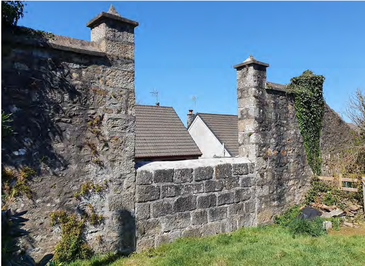
The grand entrance gateway to the Ponsanooth saltpetre refinery, supplying one of the main constituents of gunpowder to the Kennall Vale works, part of the secure perimeter wall that survived when the works were demolished in the later 20 th century and replaced by a housing estate.
