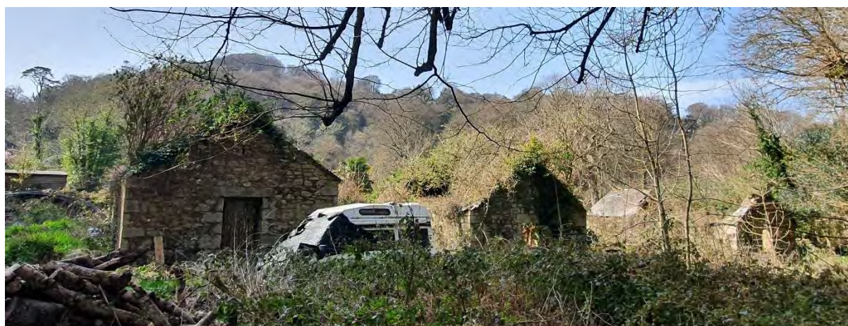
The three Kennall Vale gunpowder stores, all Listed and Scheduled. That on the left (first recorded on the 1878 OS map) is later than the other two (on 1840 Tithe Map). Each has ventilation slits on the side walls and a door at each end. All internal fittings including floors have been removed (Marilyn Ferris, pers comm).
