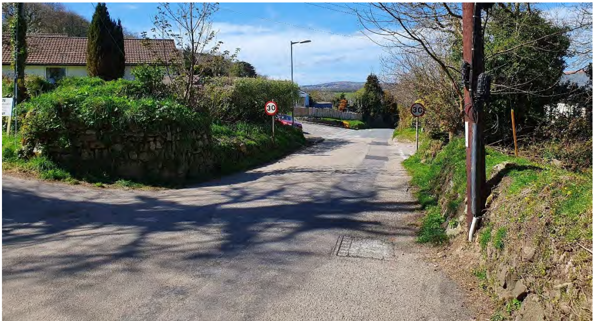
The earlier, possibly originally medieval, version of the highway from Penryn as it approaches Ponsanooth from the south and is about to descend the stretch now called Commercial Hill. A thoroughfare, designed to be wide enough, just for wheeled vehicles to pass, and with Cornish hedges still marking some of its boundary. In the distance is the rounded hill of Carn Marth, standing above the road's destination, Redruth.
