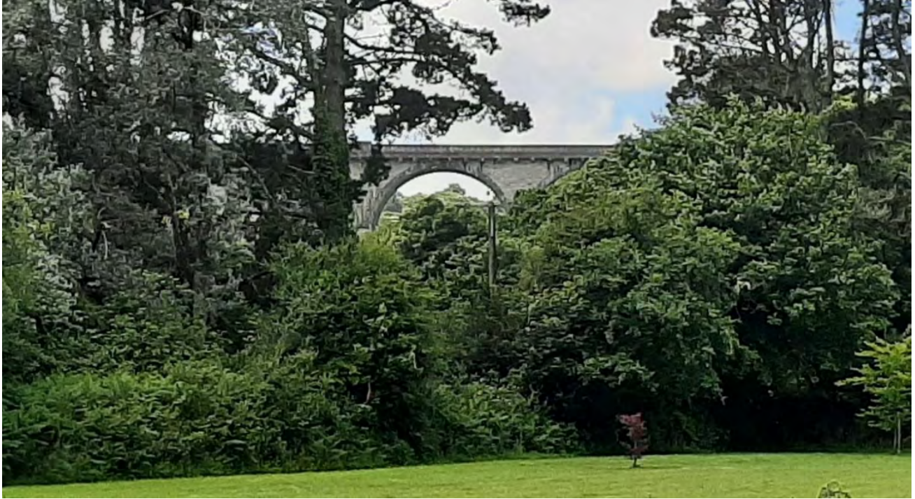
19. Ponsanooth Viaduct from Blankednick Lane (from 30 yards into farm lane
