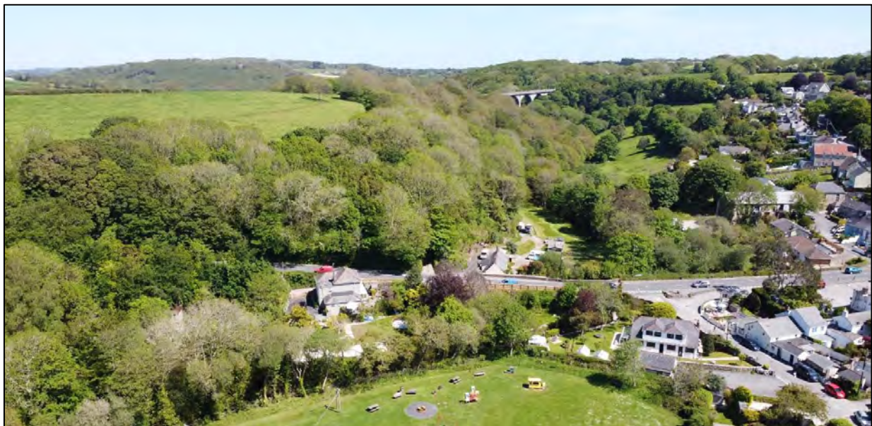
Figure 45 Kennall Valley as river flows under the listed road bridge in Ponsanooth, with viaduct in the background
