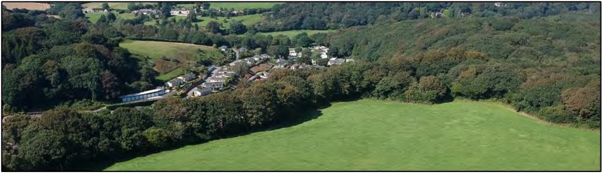
Figure 65 Cosawes Park Homes situated in the small, steep sided valley running to the north-east
