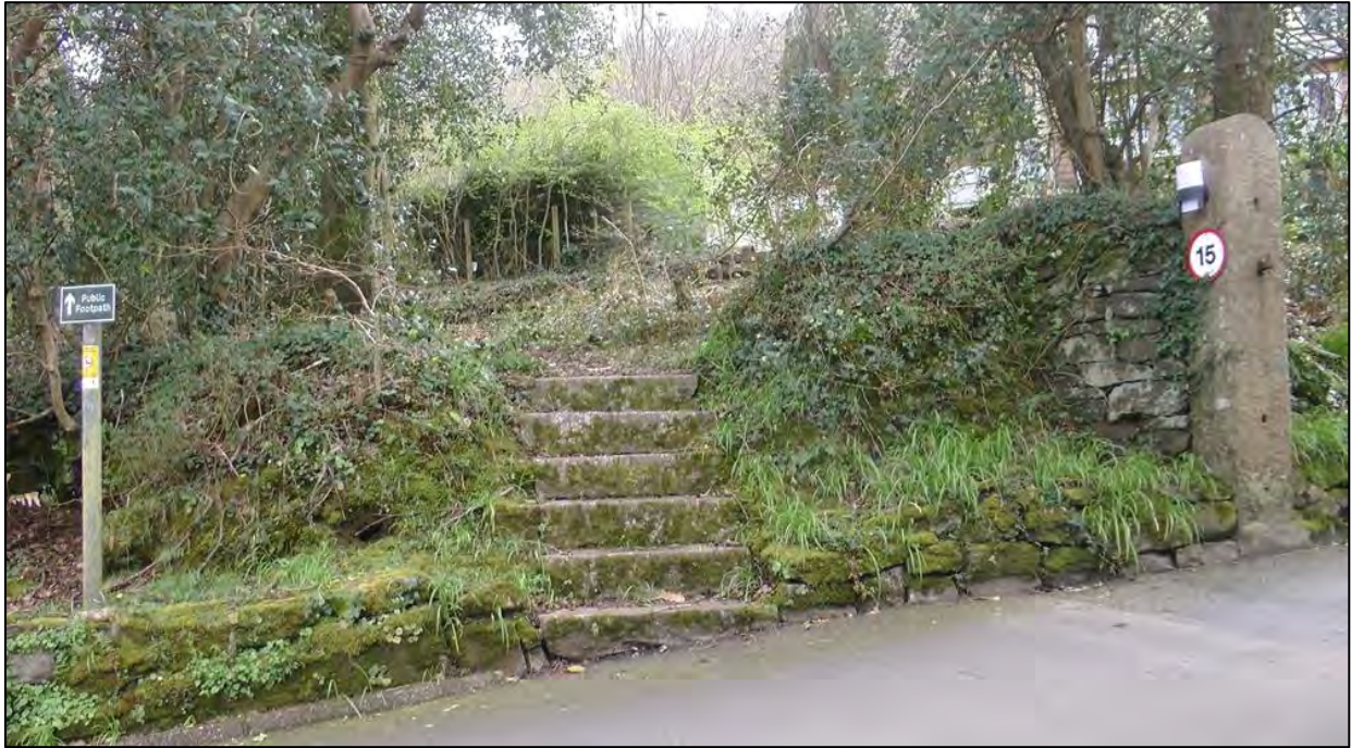
Figure 53 Granite steps to footpath from Cosawes Park Homes entrance that runs eastward at the
