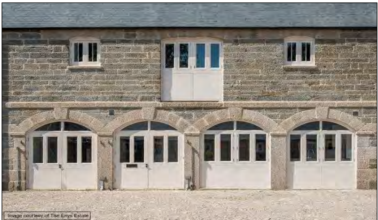
Figure 34 Enys, façade of restored courtyard building
