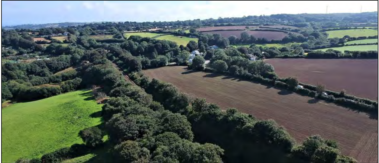
Figure 41 Railway line and A393 running parallel to each other towards Burnthouse
