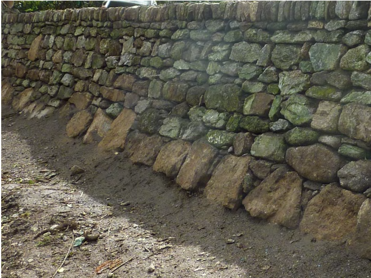
Figure 31 Repaired Cornish stone hedge
