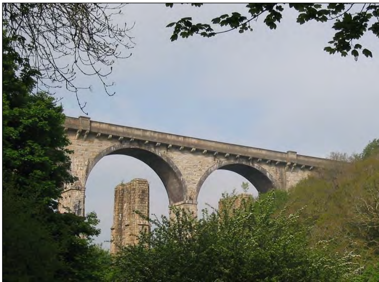
Figure 55 Viaduct from southeast
