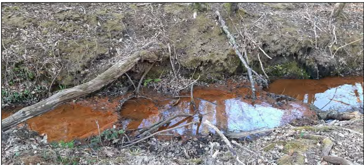
Figure 59 Drainage channel containing stagnant water
