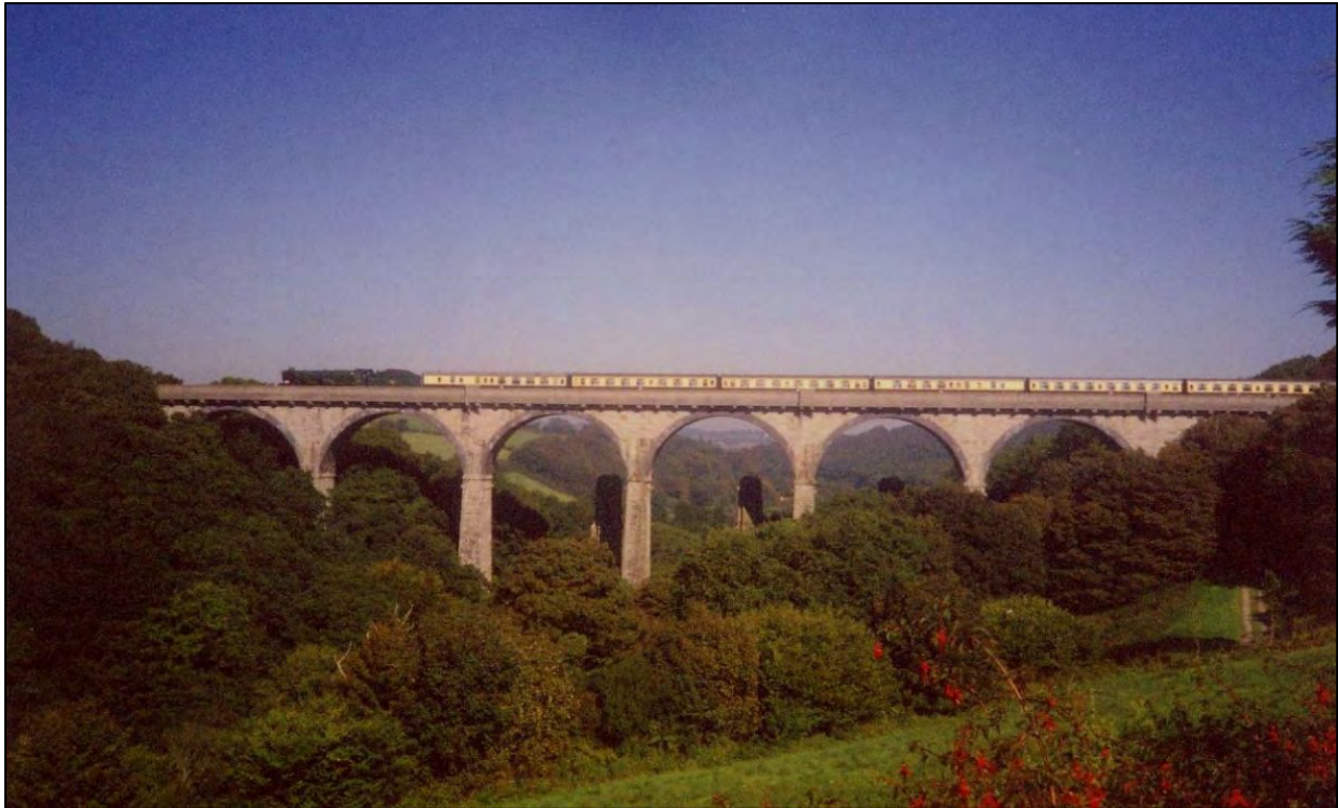
Figure 46 The Truro to Falmouth railway line viaduct, original Brunel bridge piers visible underneath.
